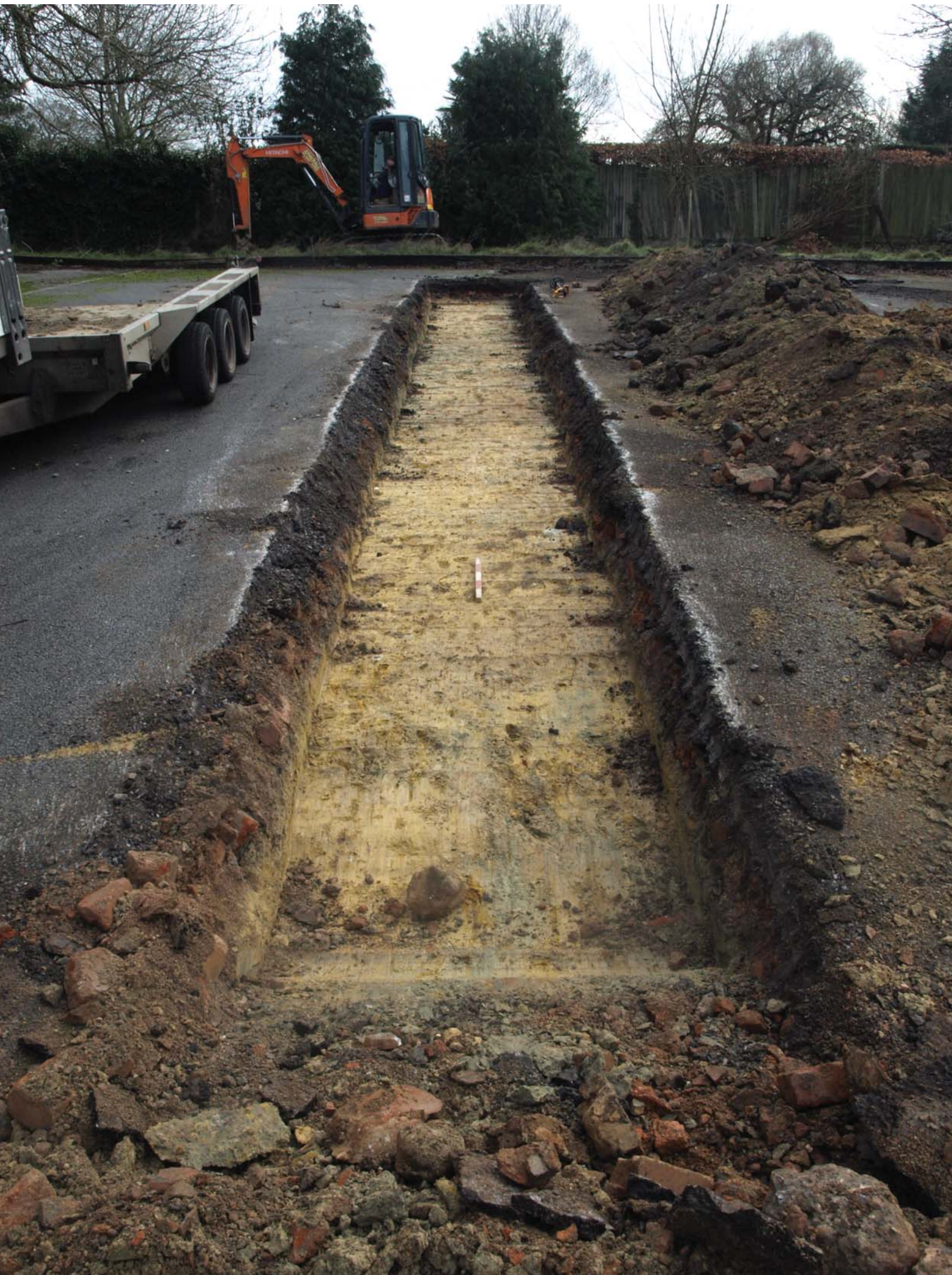
Plate 3: Looking east at Trench 1
